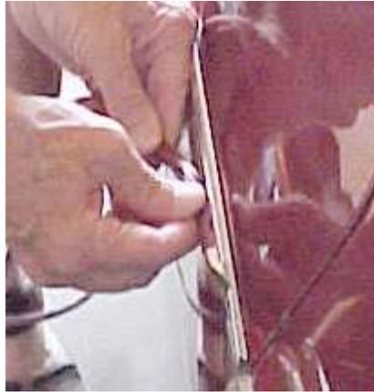
**Figure 3 Installing the vinyl insert**
